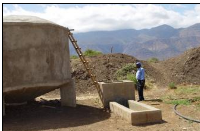
Photograph 8: A water tank and water trough for livestock built adjacent to a charco dam in Kwesasu village in the lowlands of the western Pare Mountains (photo by F. Rwehumbiza, June, 2004).
