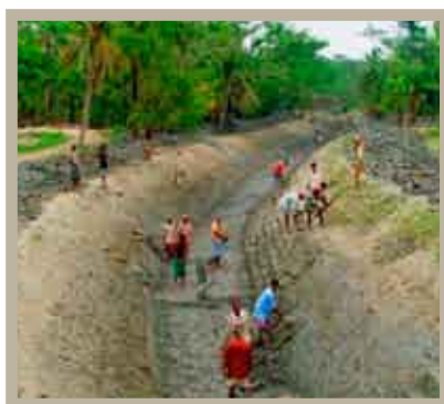
Re-excavation of the canal in Jelekhali village, Bangladesh
