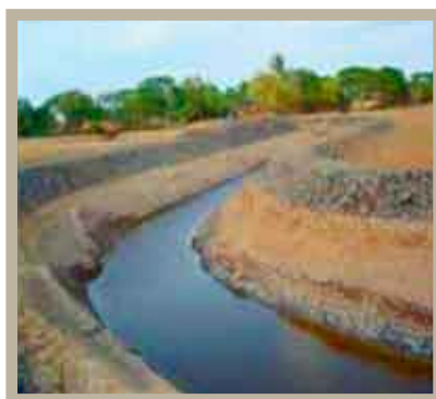
The re-excavated canal now provides saline-free water for small-scale fish culture and irrigation
