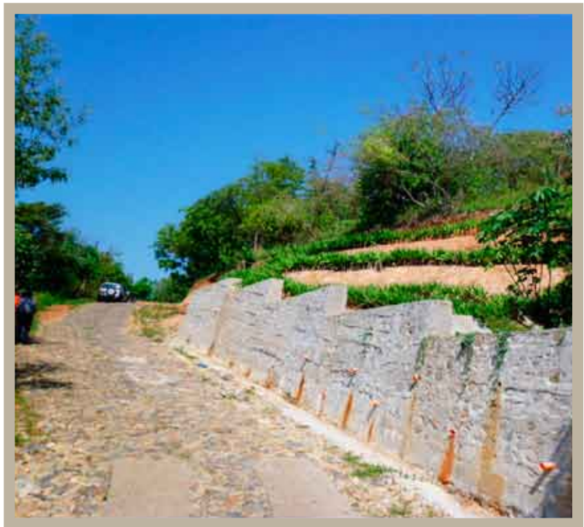
Slope stabilisation demonstration project using vegetated terraces
