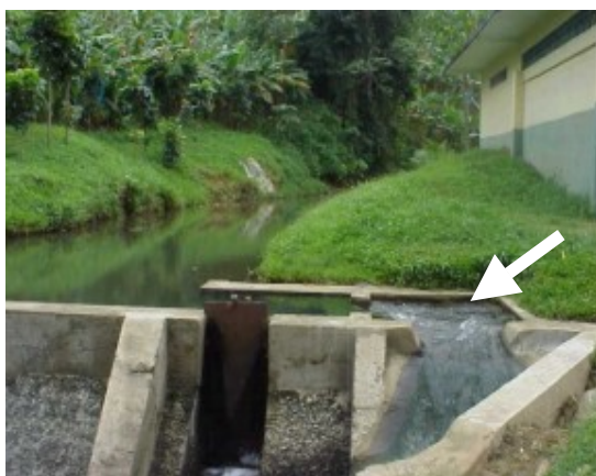
Figure 2: Talvan intake (abstraction location indicated by arrow; pump house at right; note bananas on riverbank)
