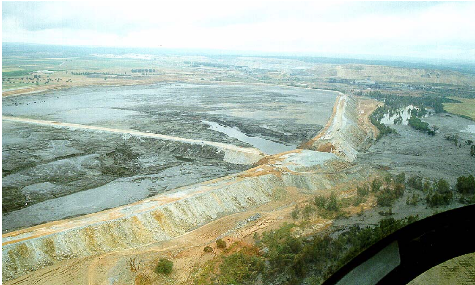
Aznalcollar Tailings Dam Failure
