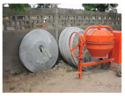
The round dome-shaped slab that was designed in Mozambique in the 1980s to cover the pit of a dry-pit latrine. The conical dome shape is strong and eliminates the need for steel reinforcement. It is the only specially designed element in the latrine programme.
