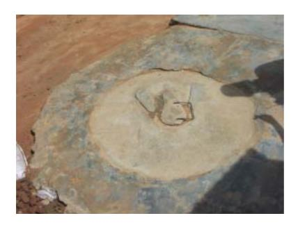
Despite the lack of water, some residents prefer to build pour-flush toilets. The round domeshaped latrine slab can be adapted for use as a cover for the septic tank.
