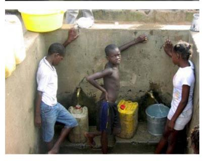
DW programmes facilitate water supply through public standposts linked to the mains water supply. Where water pressure in the mains is low but the need for a standpost is urgent, one is constructed partly below ground level. More recent work by DW to improve mains water supply to particular areas is an attempt to reduce the problems of low water pressure, but large-scale investment is also needed to improve overall city water supply in line with the growth in population of the last 25 years.
