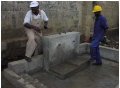
A standpost under construction. DW programmes facilitate water supply through public standposts linked to the mains water supply and constructed by teams of DW and Water Company staff. The perimeter walls reduce the amount of spillage from spreading to the surrounding surfaces. The structure is built mainly of concrete blocks or cast-in-place concrete.
