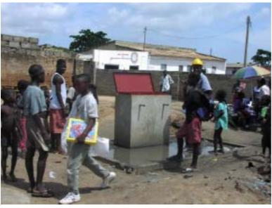
A standpost under construction. Some are being built from cast concrete rather than concrete blocks.
