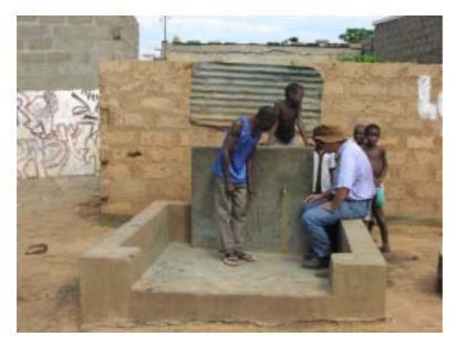
Standposts are designed to use taps that are easily available on the market in Luanda. When they break, they can be quickly replaced by the monitor chosen by the users. This has proved to be more straightforward than using special, heavy-duty taps that are less easy to obtain when they do break.
