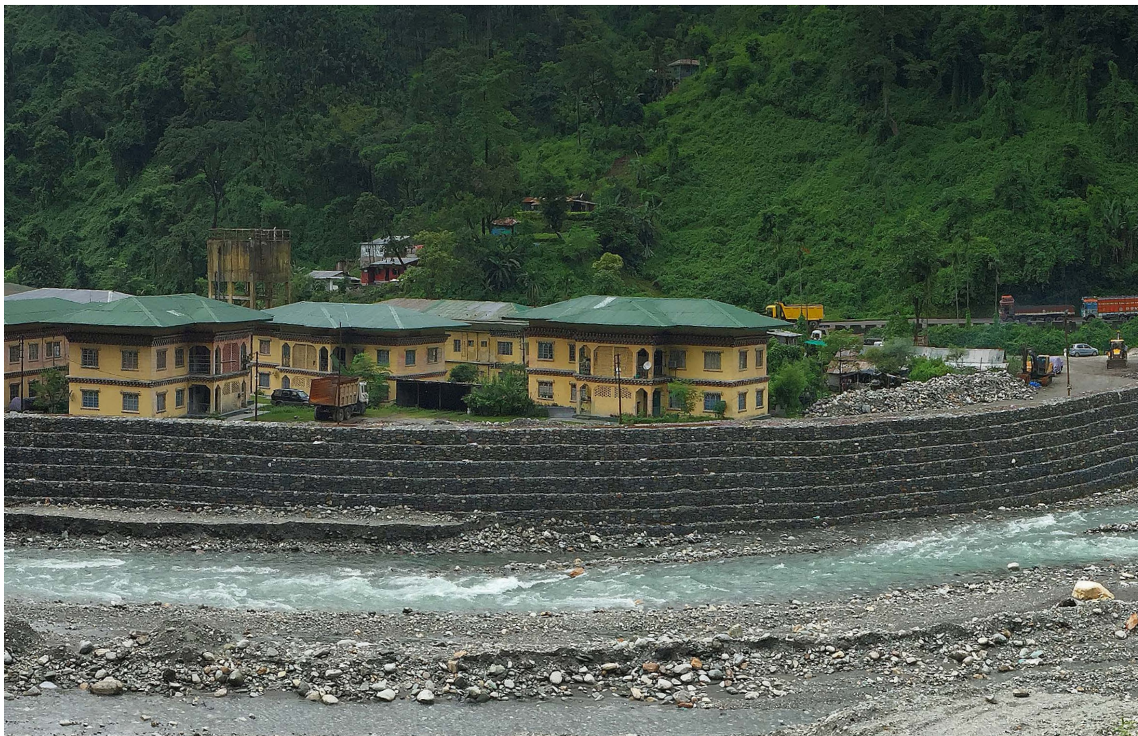
NAPA II flood protection walls, built by the Phuentsholing Municipality to protect the Pasakha Industrial zone
