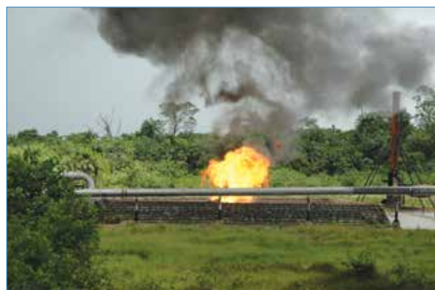
Gas flare and pipeline, Niger Delta
