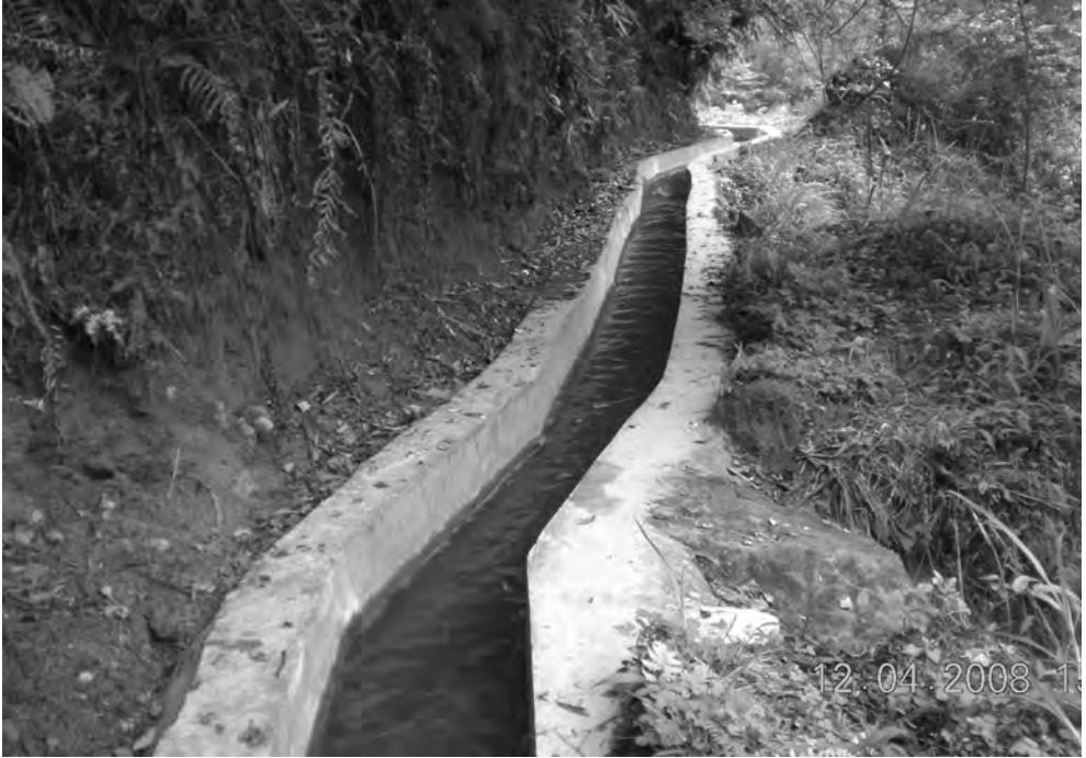
Completed ditch, Shepu Village, Naweng Township.
