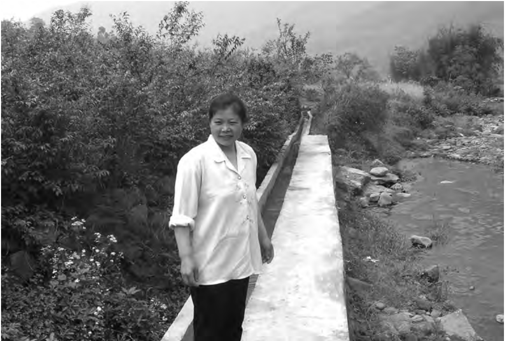
Guo Yuangui standing on the newly constructed irrigation ditch.
