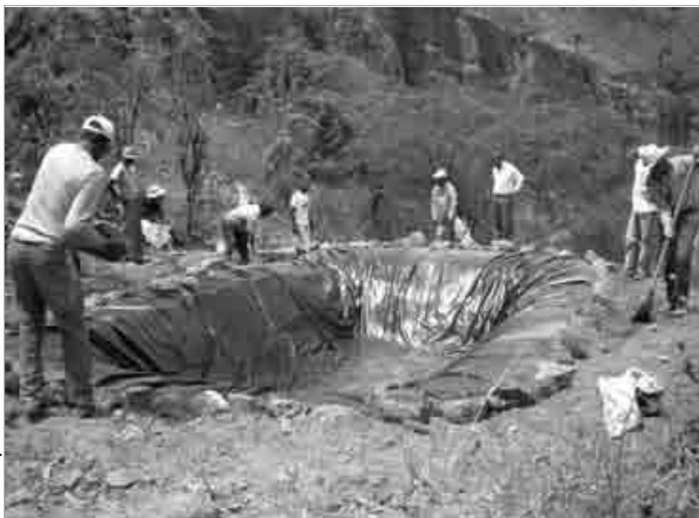
Figure 7: A minga or work party helps a colleague install his first geomembrane tank.
