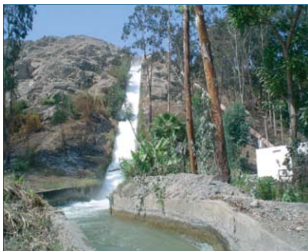
A canal and spillway at the Santa Rosa hydro project. The canal is cleaned regularly as part of the community benefits plan.
