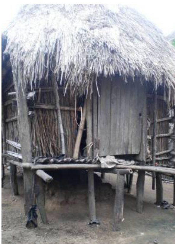
Photo 4: The main stilts are made from the trunk of Afintin trees ( Rothmania longiflora )
