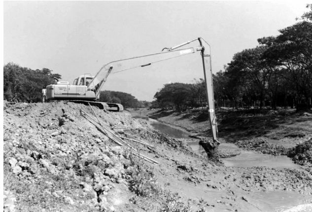
A silted-up river is dredged
