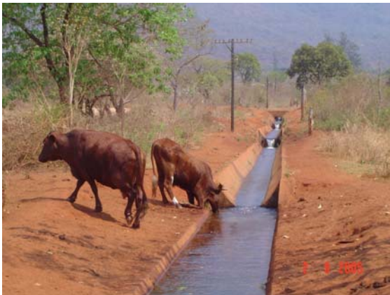
The Ga-Selati River Irrigation Scheme: a multi-use system (Photograph: R.A. Chapman)
