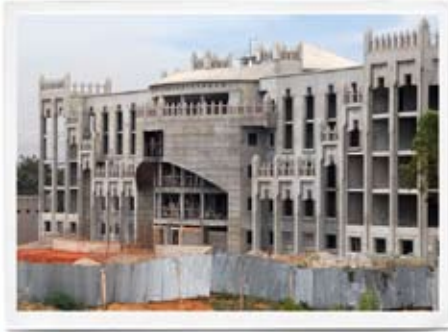
Joint Ministries Complex in Bamako under construction
