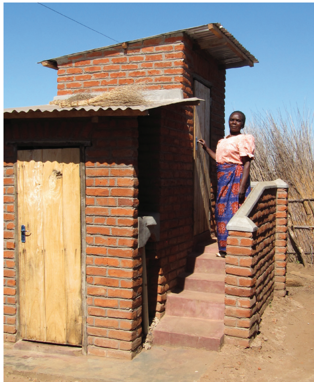
Figure 1. CCODE toilet, credit CCODE 2015
