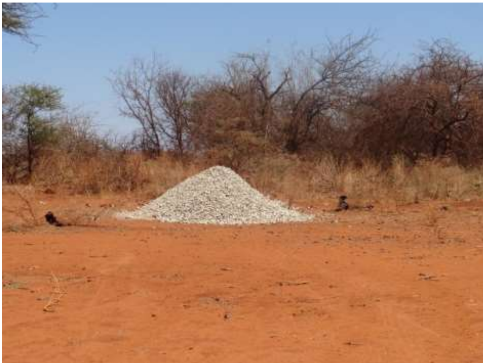
Photo 26: Construction materials at Harr Buyo water pan site
