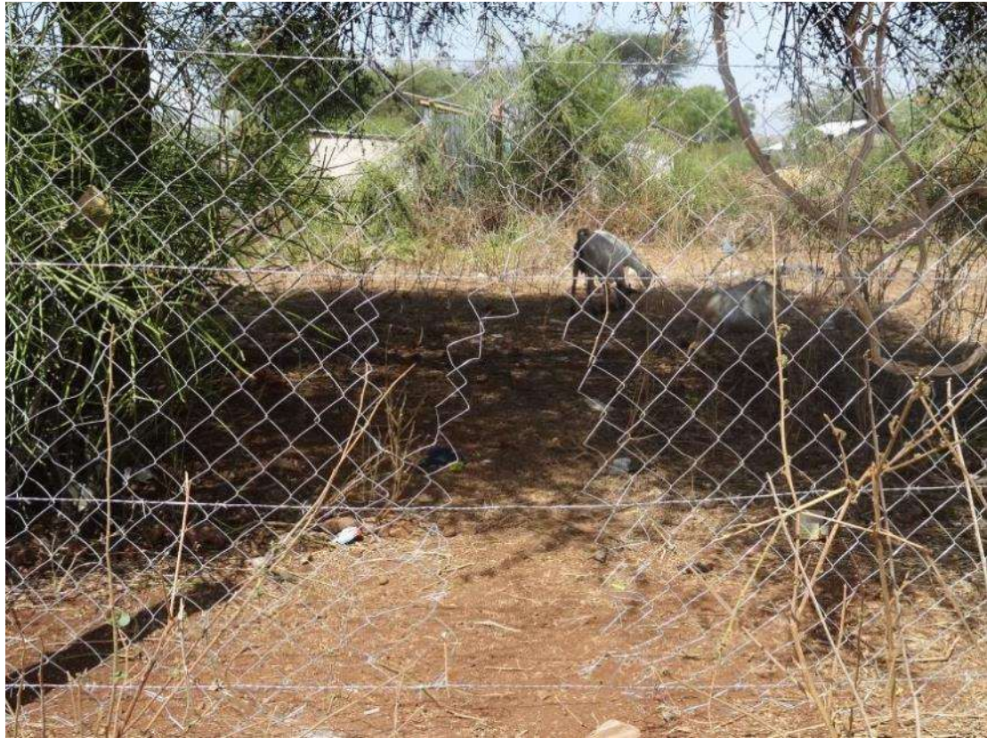
Photo 23: Hole in laboratory fence
