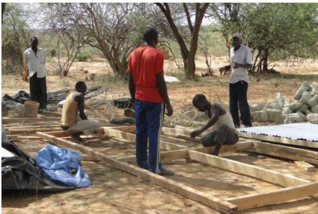
Photo 9: Workers setting up at the water tank site
