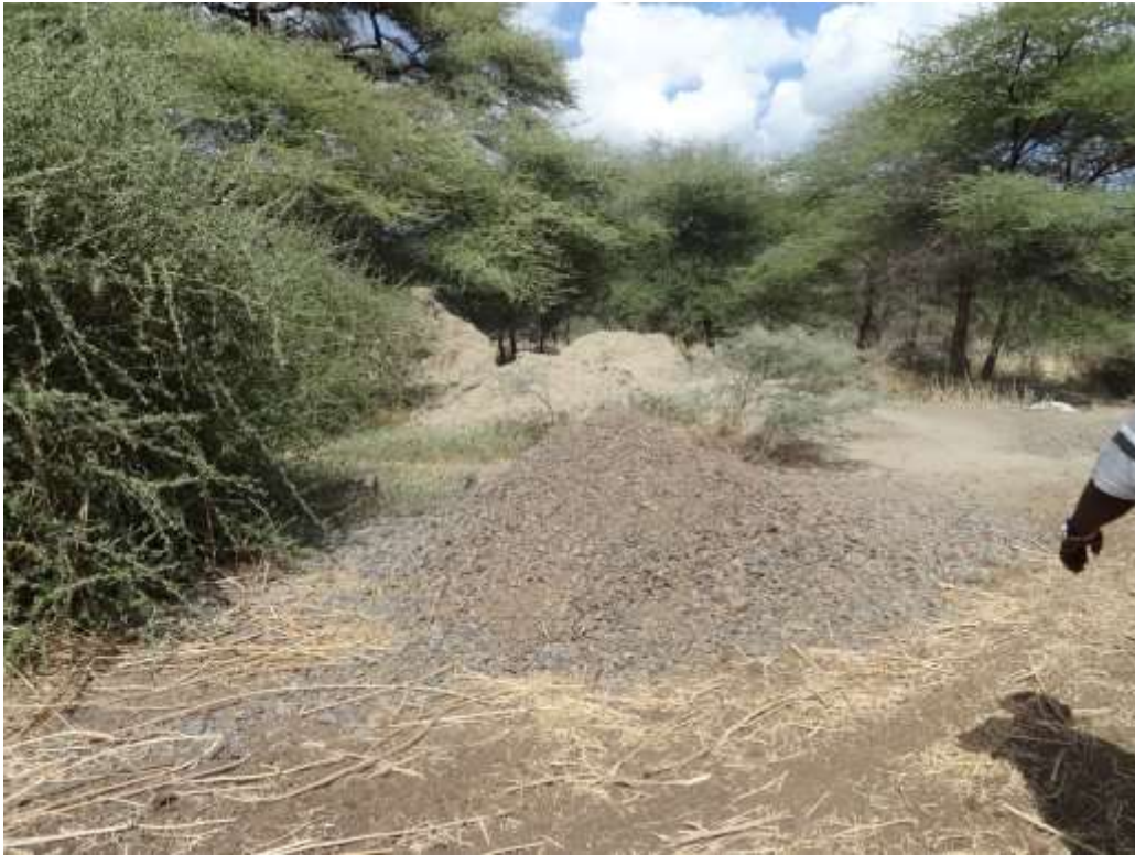
Photo 34: Construction materials at Hawaye
