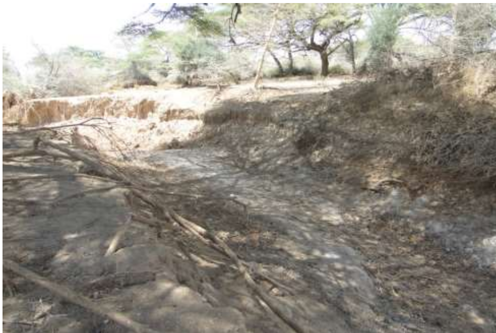
Photo 16: Spillway of Yamicha water pan
