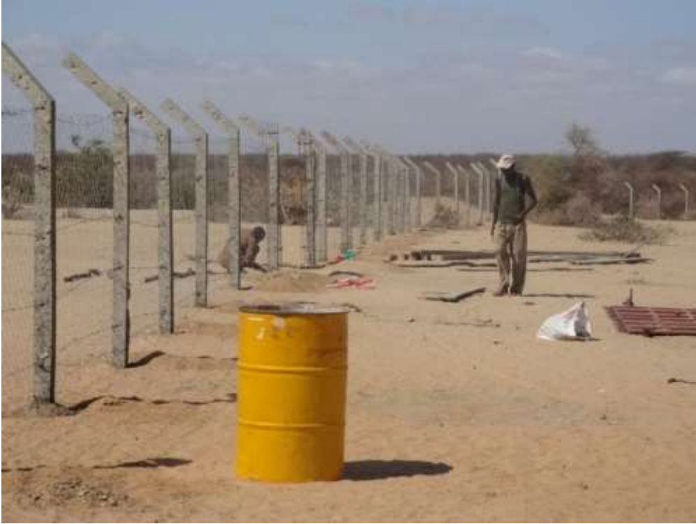
Photo 30: Fencing at Manyangap pan
