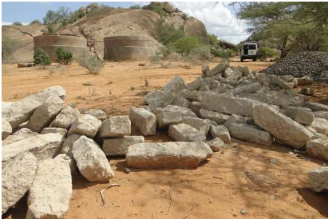
Photo 8: Construction materials at the water tank site
